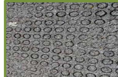
Plastic reinforcing grids (PG) filled with gravel
