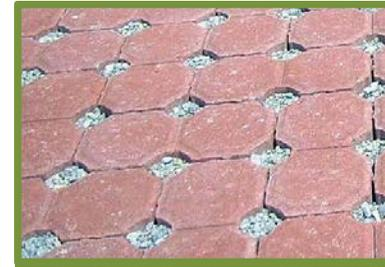
Permeable interlocking concrete pavers (PICP)
